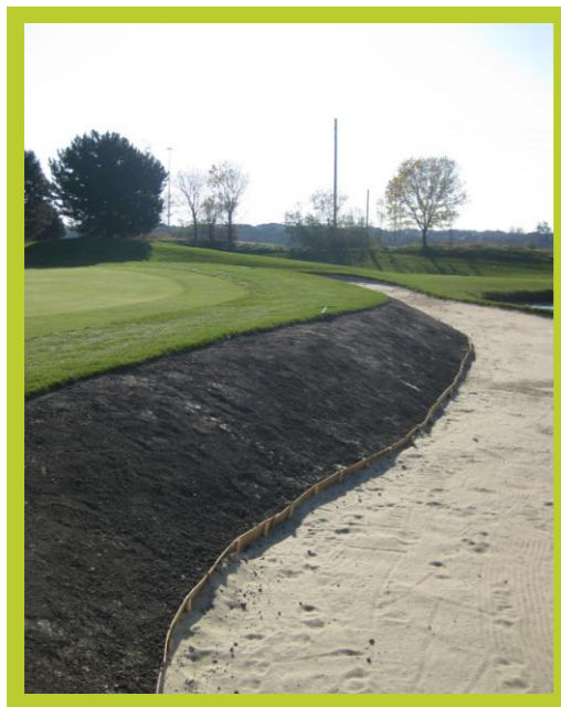
9 th Hole greenside bunker re-facing
