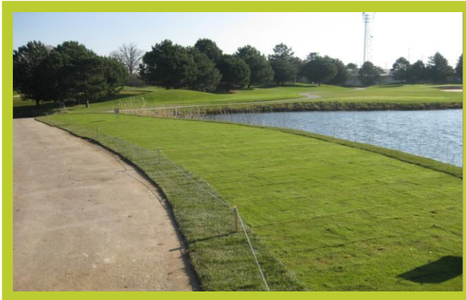
9 th Hole white tee deck re-leveling and resizing
